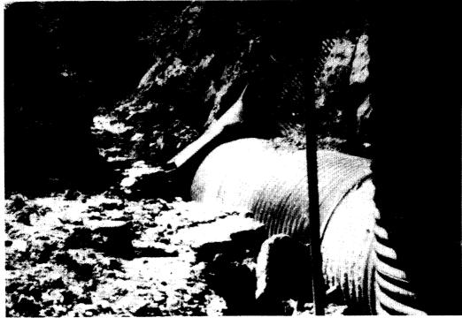
Detail of above, looking downstream along pipe from riser. Note collapse of 14-foot square anti-seep collar and the near vertical trench wall parallel to pipe in center of picture.
