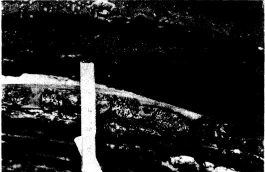
Many structures had poor joints, with large gaps between pipe sections that allow embankment soil to wash into the conduit by seepage flow. Sinkholes in fill above such joints indicates severe damage has occurred, and integrity of dam is jeopardized.
