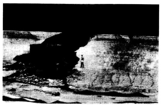
Complete failure of 25 foot high dam for "dry" pond, viewed from the pool area. The structure does not normally impound water. The 72-inch barrel pipe was apparently installed in a vertical trench cut through nearly completed embankment fill. Failure occurred during a storm that filled pool to just below enlarged top of riser.
