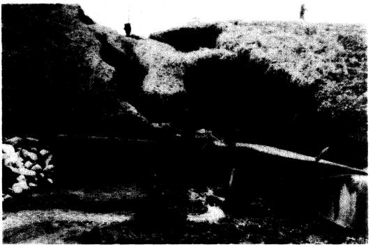
Complete failure of 25 foot high dam as viewed from downstream end of 54-inch pipe. This pipe was apparently installed in a vertical trench cut through partially completed embankment fill. Loss of soil support due to piping of surrounding backfill resulted in collapse of pipe and catastrophic release of flood waters.
