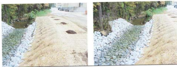
Pictures showing upstream portion of the Goodwin Run Sinkhole repair.
