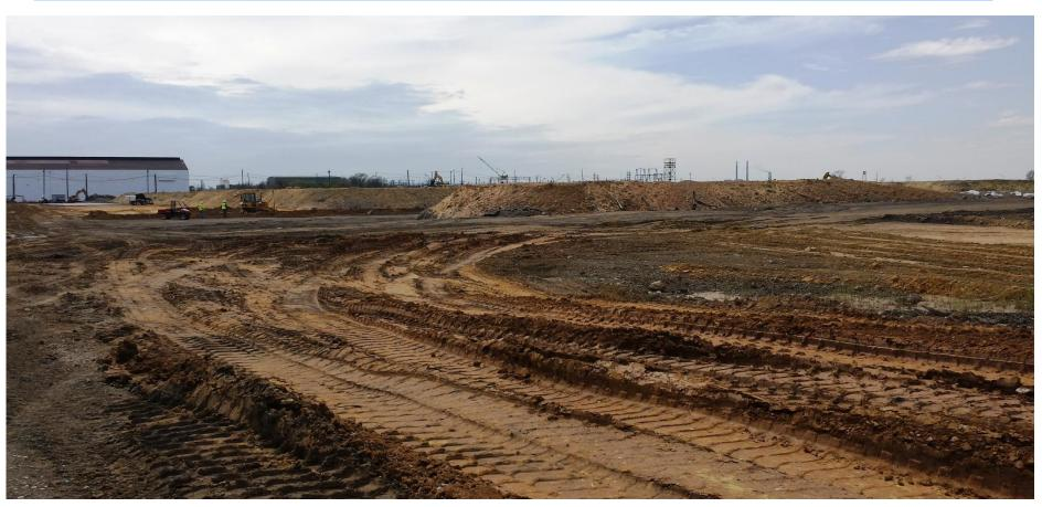
Surcharging Process recently completed Excess clean soil to be relocated prior to building construction
