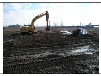
PHOTOGRAPH 10 Backfill of Southern Trench
