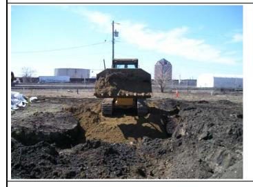
PHOTOGRAPH 7 Backfill of Central Trench
