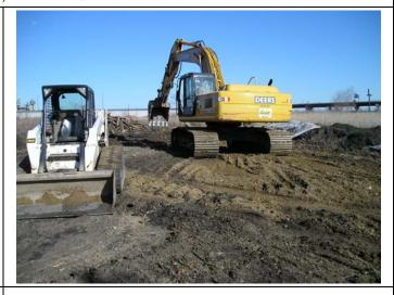
PHOTOGRAPH 8 Compaction of Central Trench
