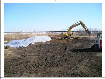
PHOTOGRAPH 4 Compaction of Northern Trench
