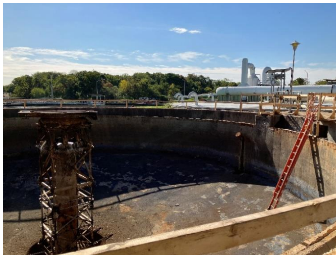
Image 02: GBT #2, Under construction.
