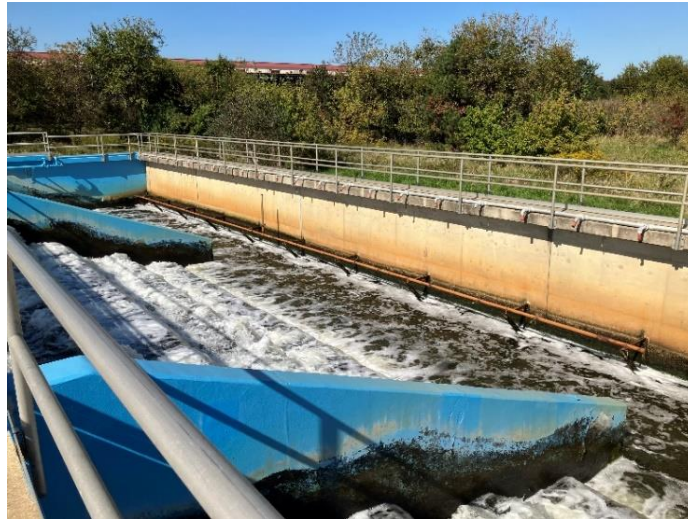
Image 05: Step Aeration system, final effluent.
