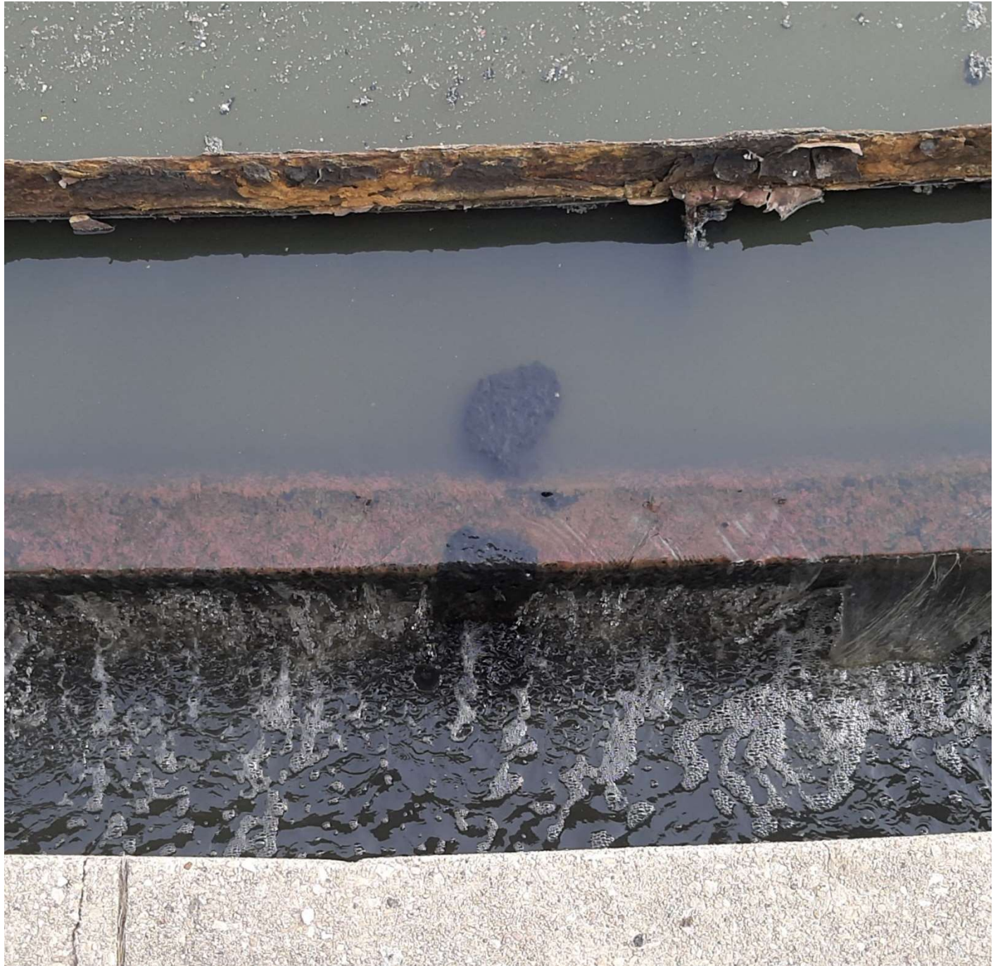
12/14/22 PST #1 solid masses overflowing the weir
