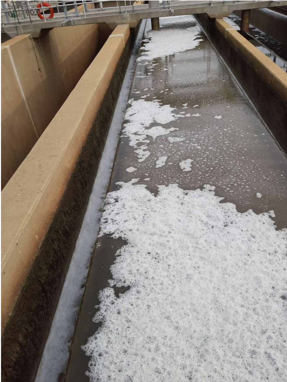
12/14/22 DNF during a “bump” cycle used to release nitrogen gas trapped in the filter causing temporary foaming during the process.
