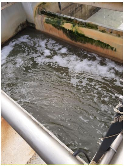
Final effluent overflow point- grey effluent with slight foaming due to turbulence. 1/31/22
