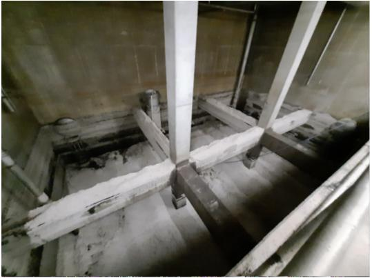
10/6/2021 In the backwash chamber- filter media on center horizontal beam
