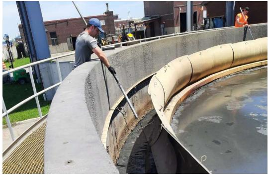
5/18/22 operators cleaning the solid particles that are accumulating on the weirs of the GST #1.
