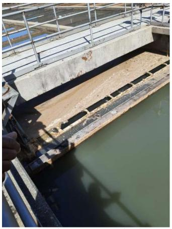
5/18/22 scum and FOG at scum trough. When rotated the scum trough will collect the FOG and scum
