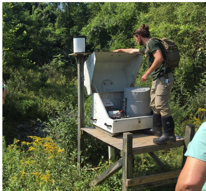
Figure 9c. FRCO's outfall monitoring storm box in August 2019.
