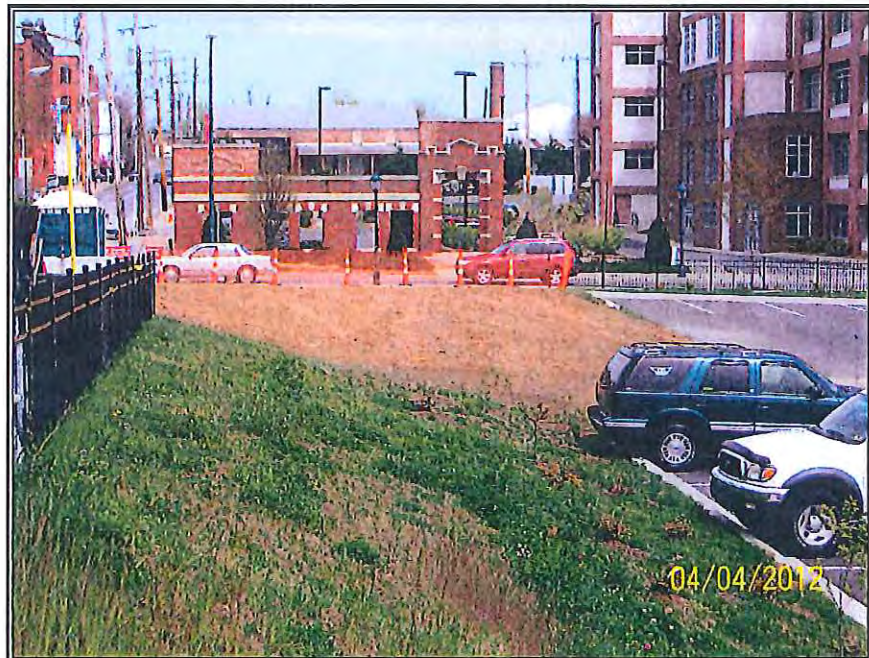
149 West Franklin Street (After)
