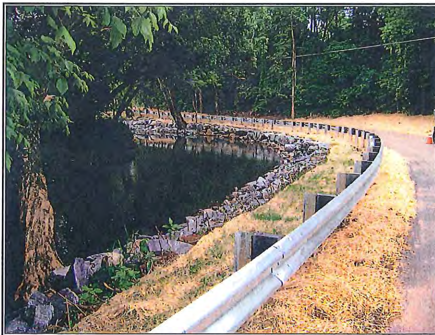
Stream Bank Restoration (After) Lehmans Mill Road Washington County Engineering & Construction
