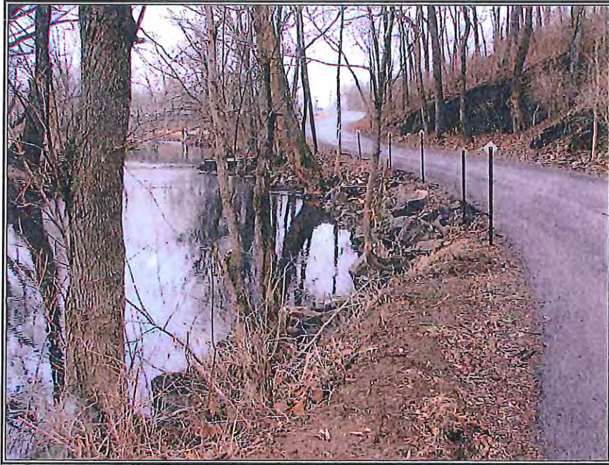
Stream Bank Restoration (Before) Lehmans Mill Road Washington County Engineering & Construction
