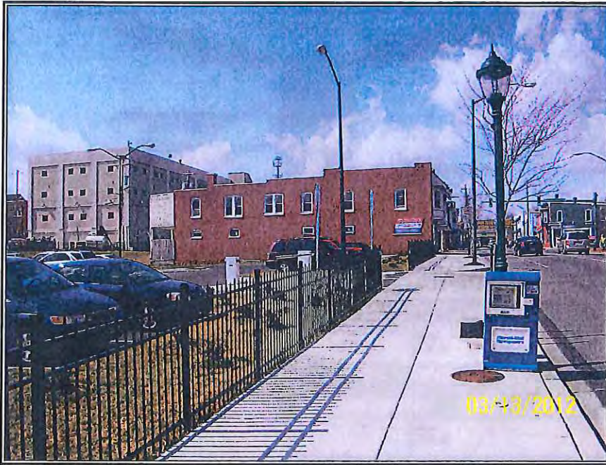
149 West Franklin Street (Before)
