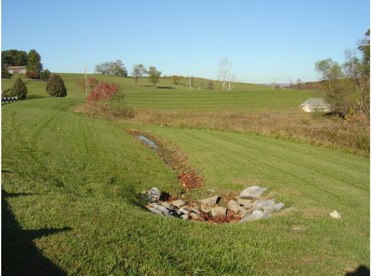
Figure 37. Example of a wetland mitigation site that has been encroached upon and partially destroyed by way of mowing.
