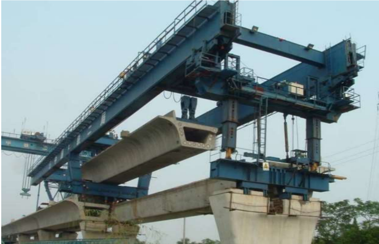
Figure 15. Full Span Launching Construction Method (Courtesy of SHCG)
