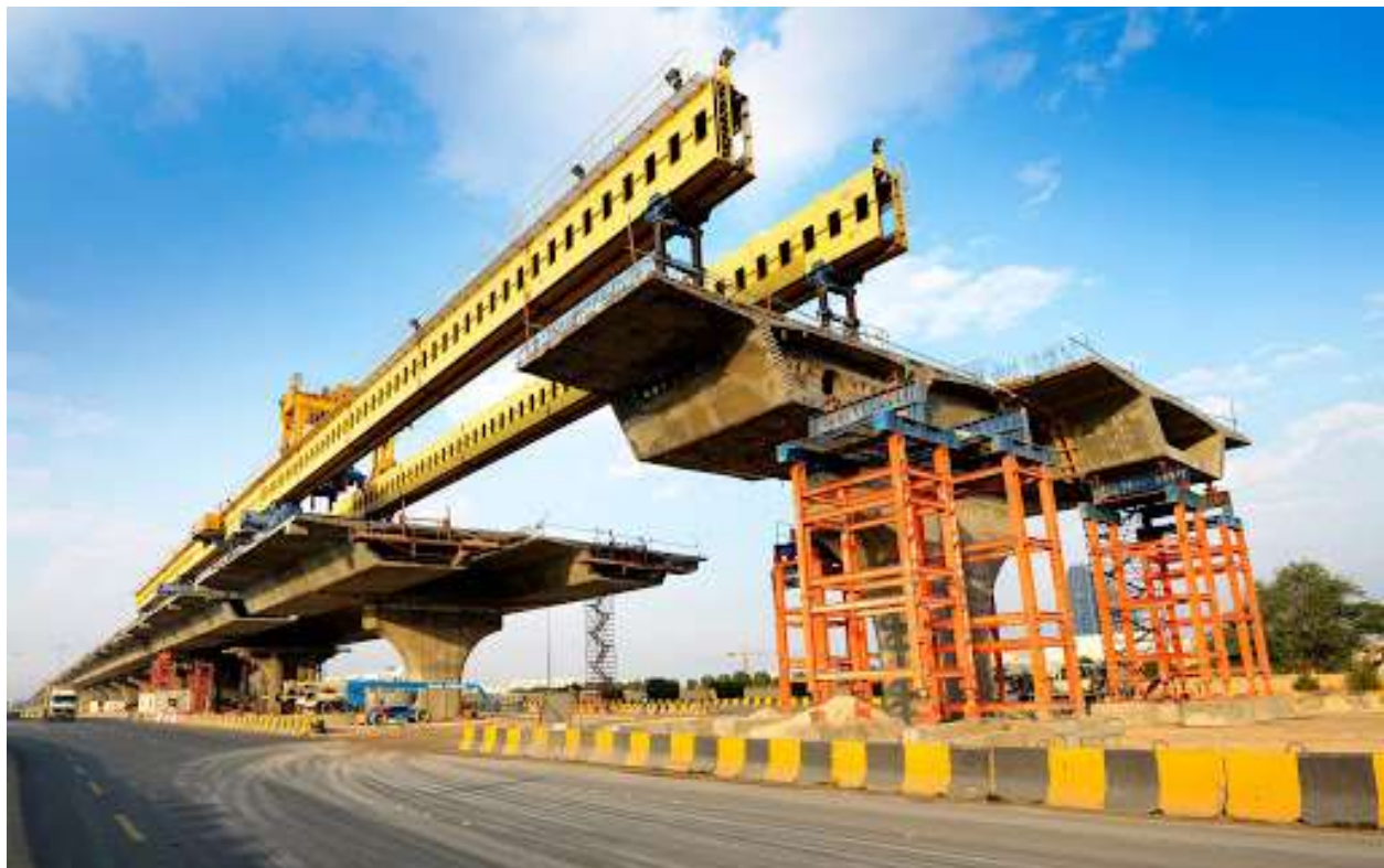
Figure 14. Balanced Cantilever Construction Method (Courtesy of WSP/Pace)
