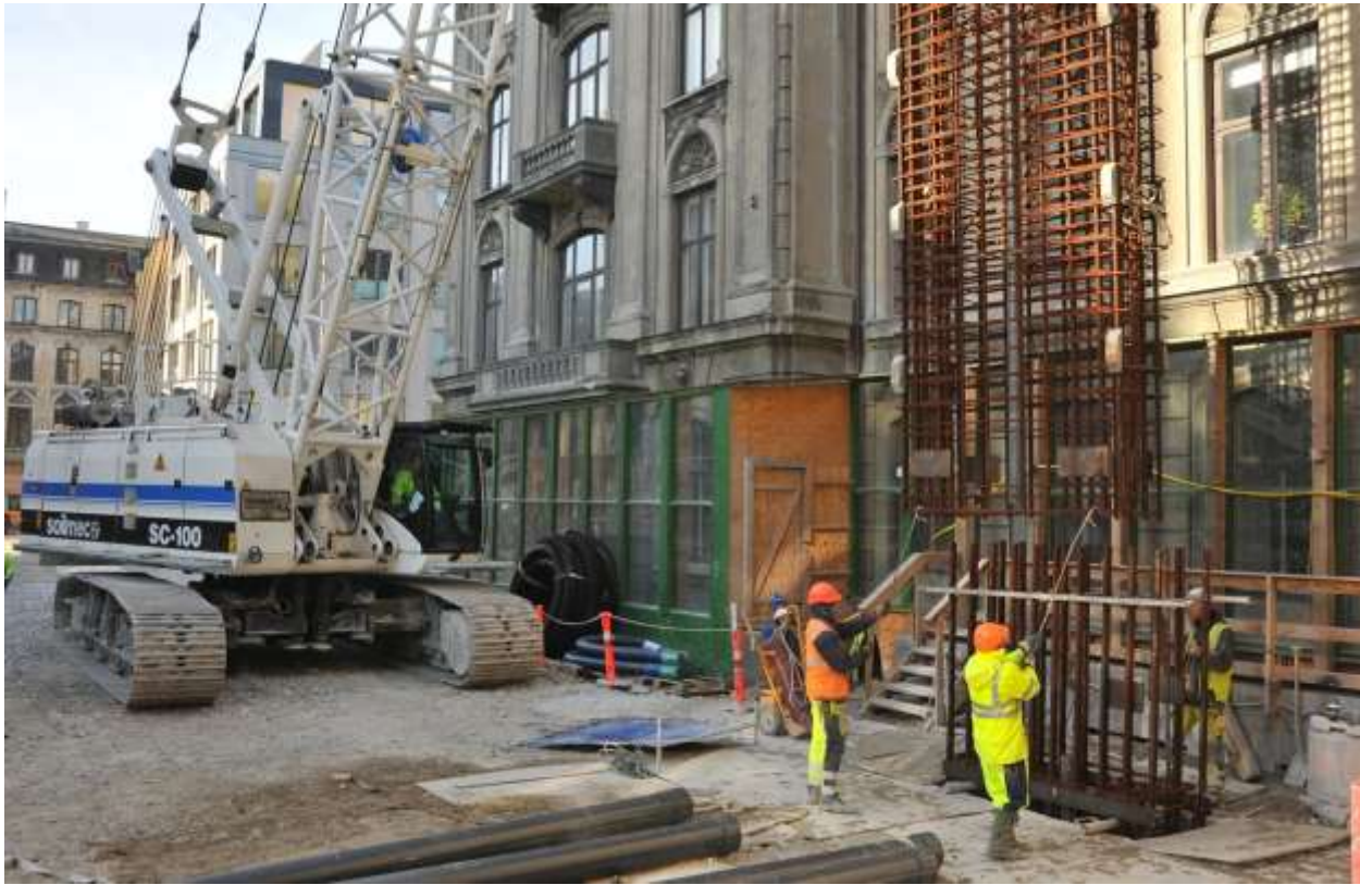
Figure 10. Installation of Rebar Cage Segments for Typical Slurry Wall Panel
