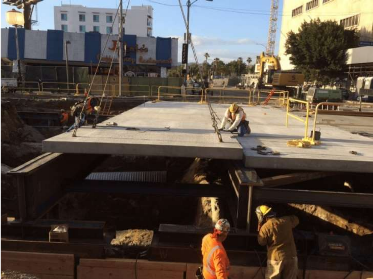
Figure 11. Street Decking (Purple Line Extension, Los Angeles, CA)
