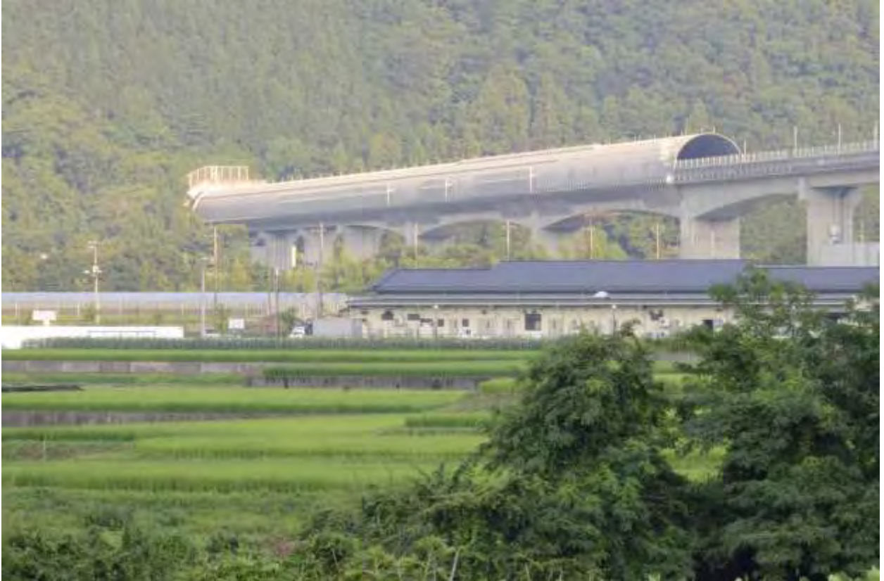
An elevated guideway emerges from a tunnel above farmland. The maglev pushes a wave of air out of the tunnel that causes noise and vibrations, so a special hood is used to more gradually vent the air. (Kevin Rector / Baltimore Sun)
