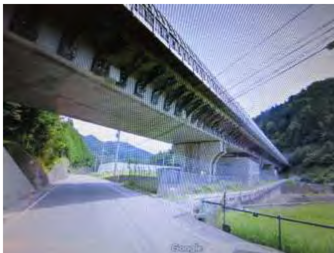
Reality - SCMagLev viaduct fencing in Japan - photo 2.
