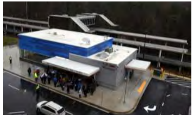
New BWI Rail Station. Photo by B. Taylor
