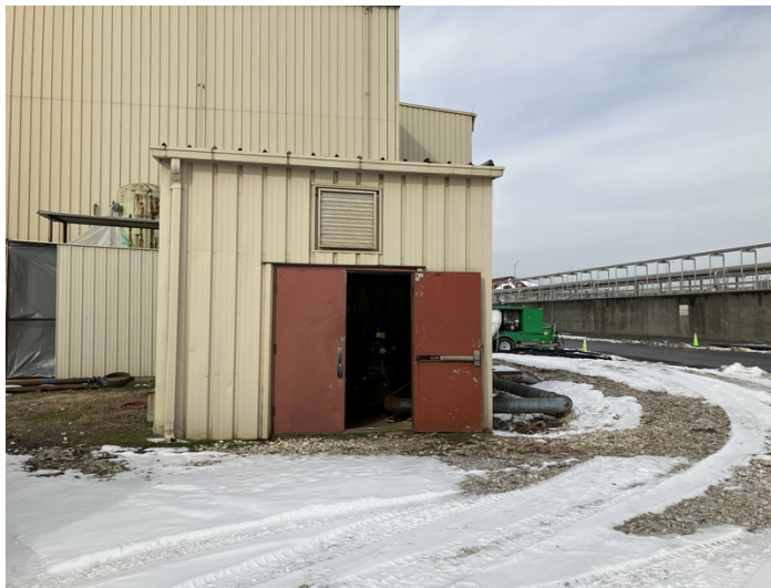
Image 05: Flushing water pit location.
