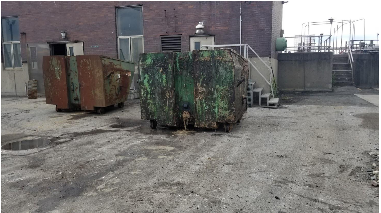
Figure 1a: A leaking hopper with FOGs by the transfer station and the northwest side of the combined influent building.
