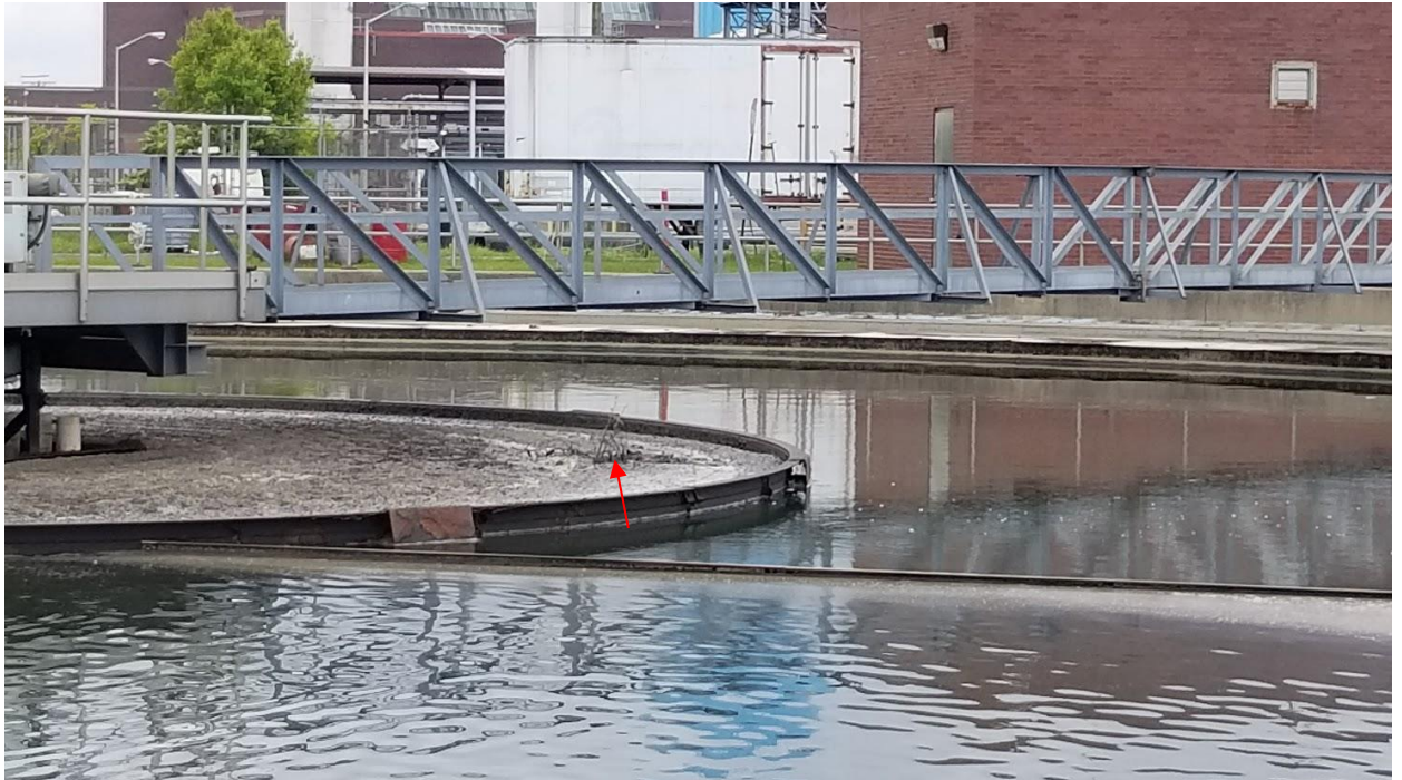
Figure 5e: Woody vegetation growing at the center/ influent side of Clarifier # 6A (pointed to with a red arrow)
